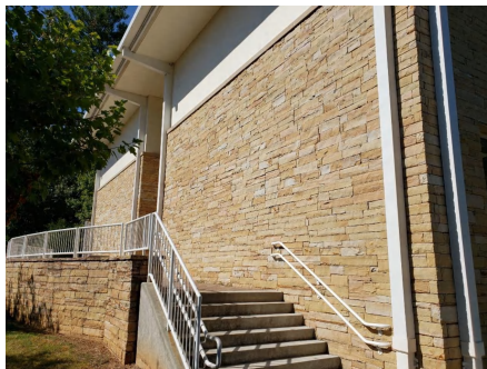
3). Southwest Elevation - Nov 22, 2019
